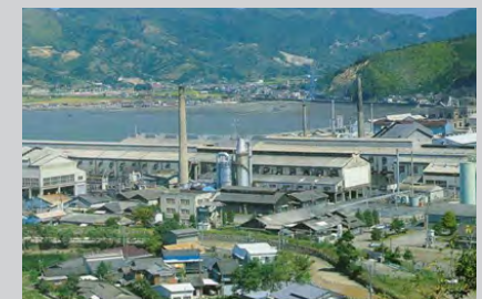
Tanoura Production Plant Iso-Static and Extruded Materials
